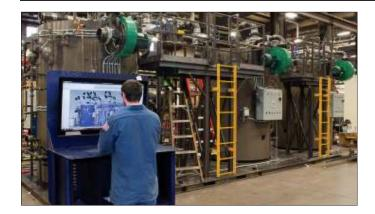
Put your project on the **FAST TRACK**. Fulton Engineered Systems include factory test fired boilers and single point utility connections significantly reducing installation resources and startup time requirements.
